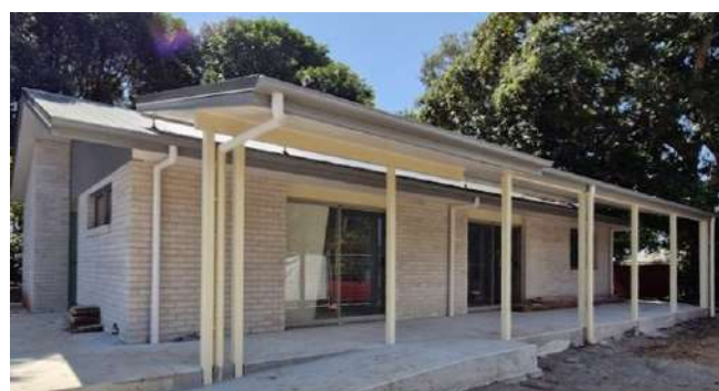
External painting completed—looking tidy
