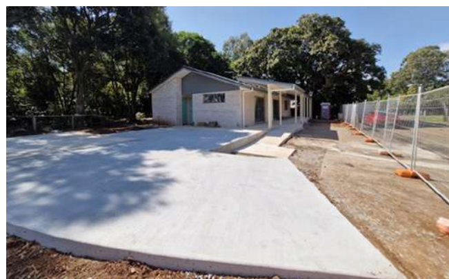
Beautiful shed slab, driveway and piazza
